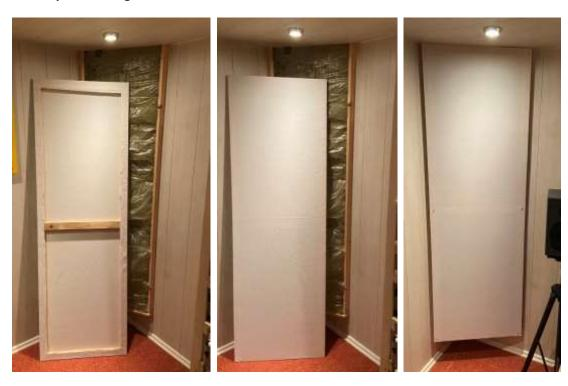
Hold the cover to the corner absorber and fasten it with 6 screws to the roof battens attached to the side of the damping elements. Tip: Measure the exact distance between the two panels and pre-drill in the cover frame with this distance. I recommend being two persons or having a good breakfast before
