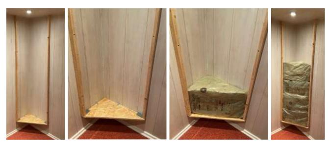
First divide the wood (MDF) panel diagonally and cut off the tips. Then screw the two roof battens to the wall at a distance of 35 and 50 cm from the corner. Attach the brackets below and screw them onto the triangular plate. Attach two additional small brackets to the wall for stabilization. Stack the triangular absorber packs up to the ceiling. Compress the packs and put one more on top to make it last.
