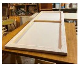
First build a rectangular frame from roof battens. Outer size:  $190 \times 65 \text{ cm}$  (If you are building the modules for a higher room, change the dimensions accordingly). I held the ends together with a  $90^{\circ}$  angle clamp, predrilled the protruding slats twice (!) and screwed the corner together with two  $4.0 \times 70$  wood screws. Insert one or two cross braces in the middle for stabilization.
